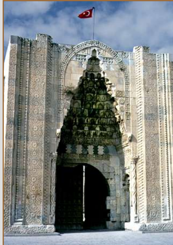
Caravanserai of Aksaray (Turkey), 1229. Financed by a waqf for use by merchants.
