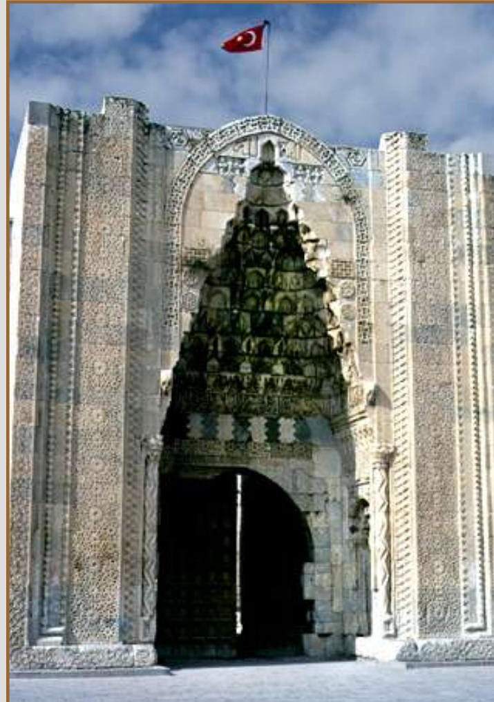
Caravanserai of Aksaray (Turkey), 1229. Financed by a waqf for use by merchants.
